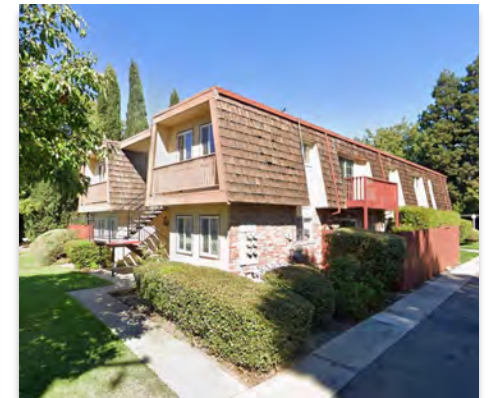
2702 Jones Road Walnut Creek
